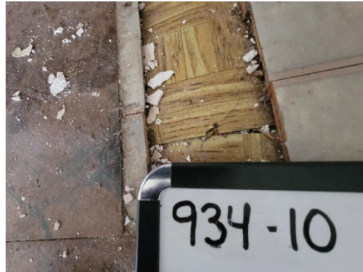
934-10 Rolled Flooring/Adhesive Interior Bathroom (Bottom Layer)
