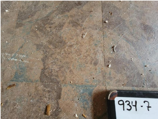
934-7 12"x12" Floor Tile/Adhesive Interior North Bedroom (Top Layer)
