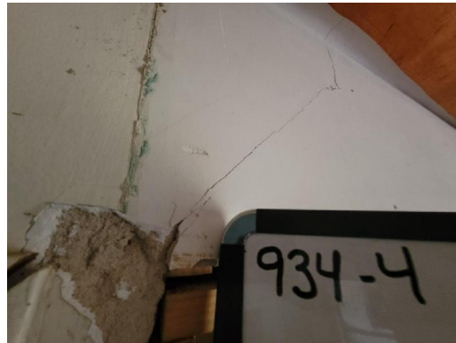
934-4 Plaster/Skim Coat/Rough Coat Typical Interior Walls/Ceilings
