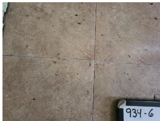
934-6 12"x12" Floor Tile/Adhesive Interior Rear Entry
