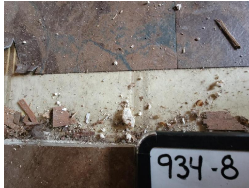
934-8 Rolled Flooring/Adhesive Interior North Bedroom (Bottom Layer)
