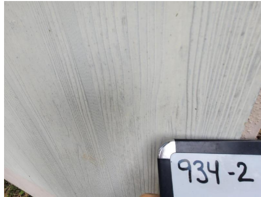
934-2 Cement Board Exterior West Wall
