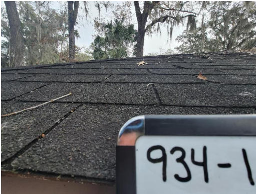
934-1 Asphalt Shingle Typical Exterior Roof
